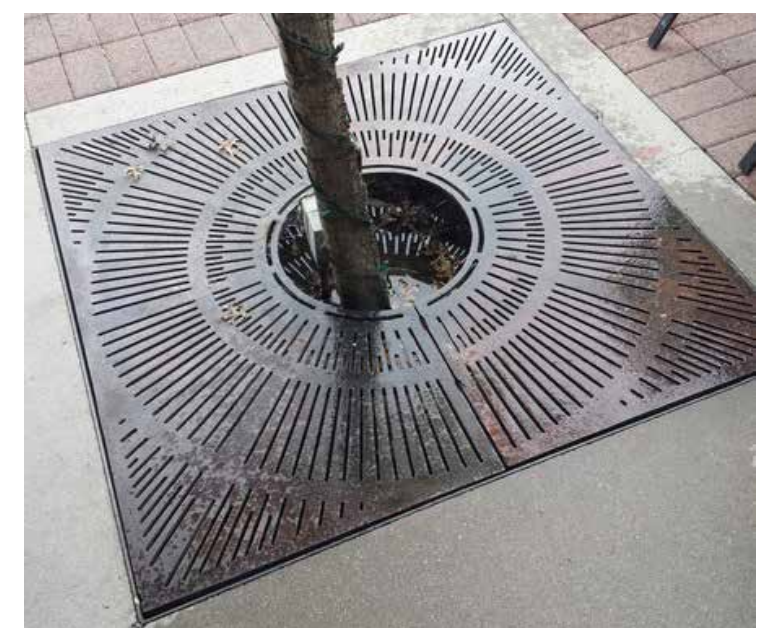
Tree Grate Mfr./Supplier: Urban Accessories Model: COHO, 4'SQ Finish: Raw Natural Finish
