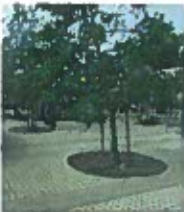
Stanford sand permeable pavers with brown w/buff aggregate bands.
