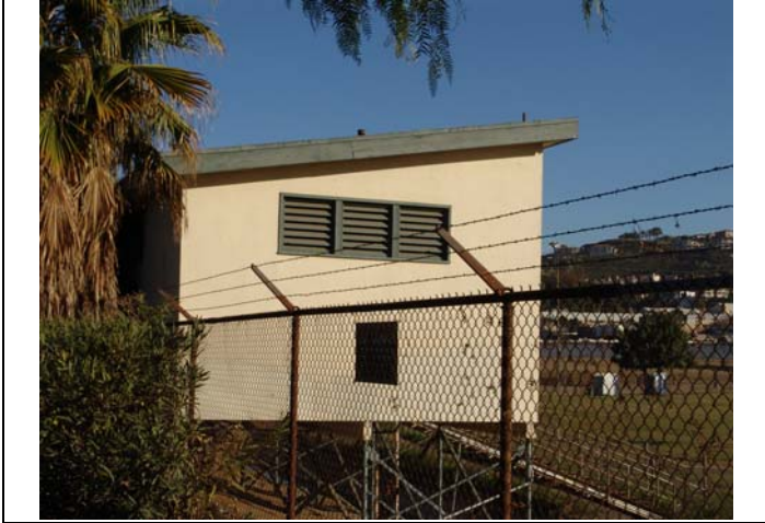
Image 1: View Facing North at South Elevation
