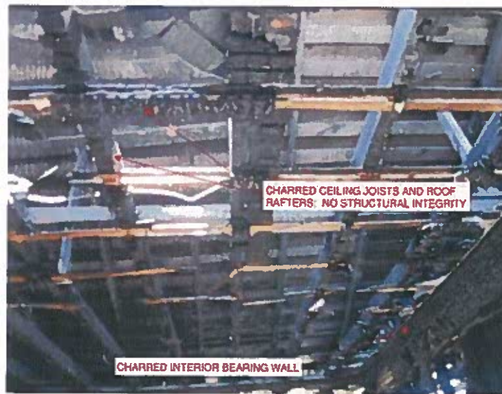
Photo 4: Interior View of Ceiling and Roof Framing
