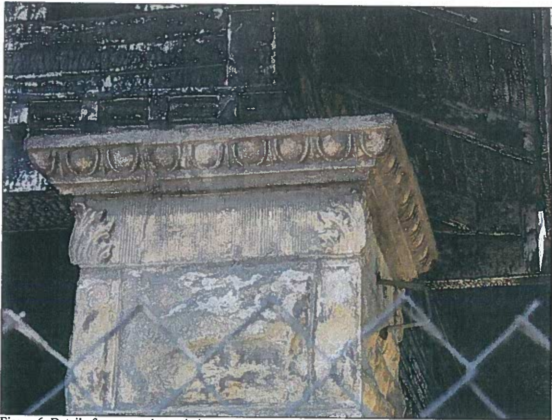
Figure 6: Detail of concrete pier capital.
