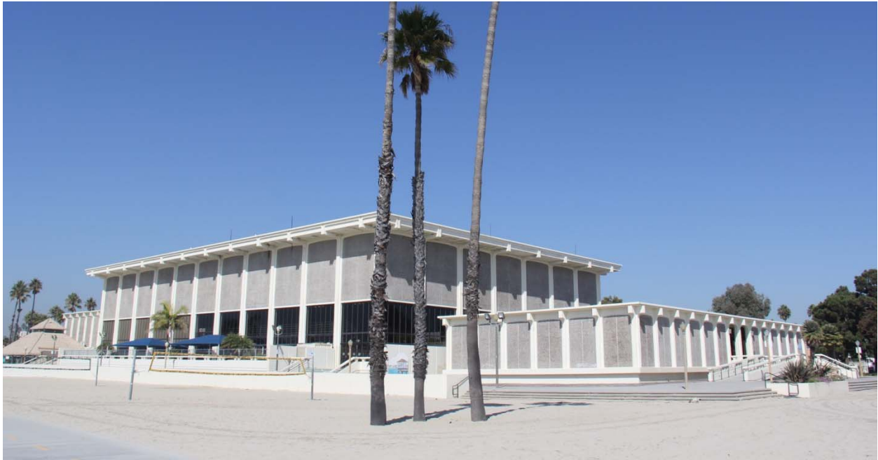
Figure 5 – Locker Building, View from Southeast [with Natatorium Building in the background]
