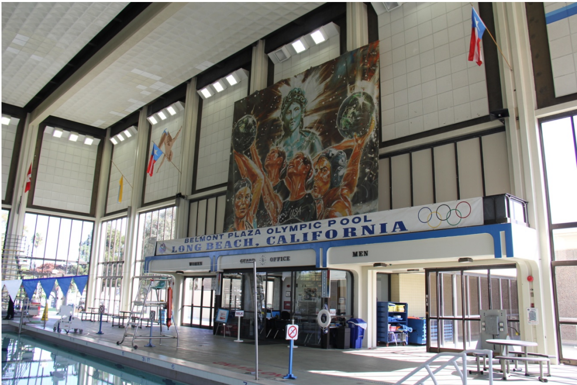
Figure 12 –Natatorium, Balcony/Entrance at East End (next to Locker Corridor)
