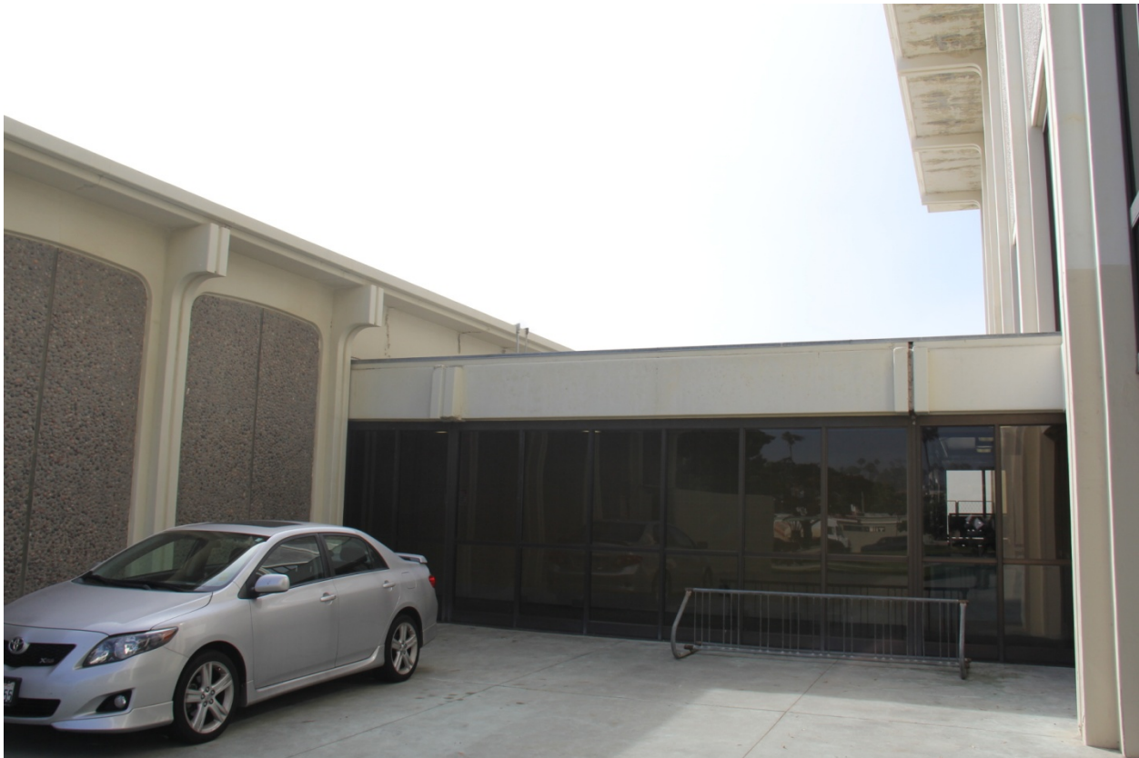
Figure 8 – Locker Building to Natatorium Connection Corridor, North View
