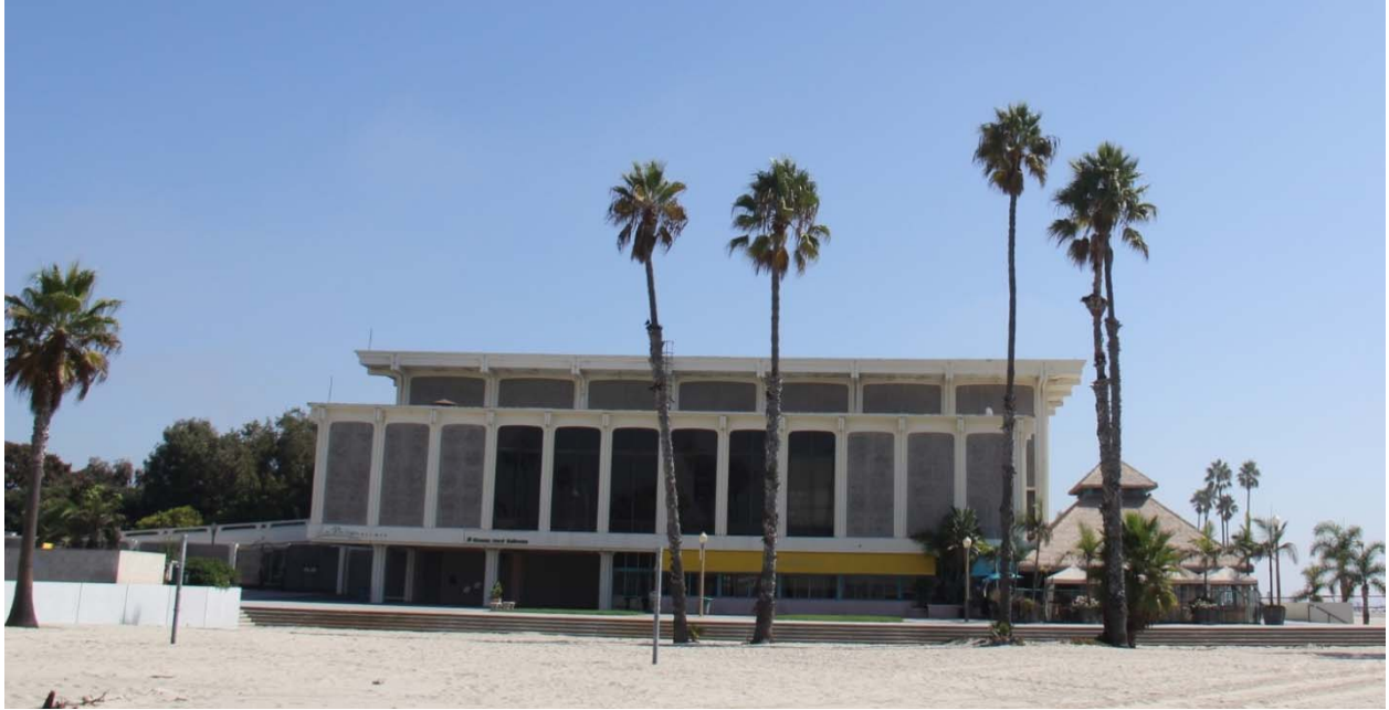
Figure 3 – Community Facility Building, View from West [with Natatorium Building in the background]
