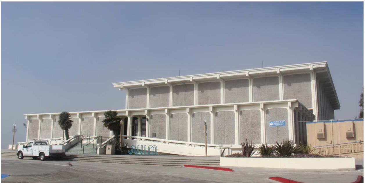
Figure 4 –Locker Building, View from Northeast [with Natatorium Building in the background]
