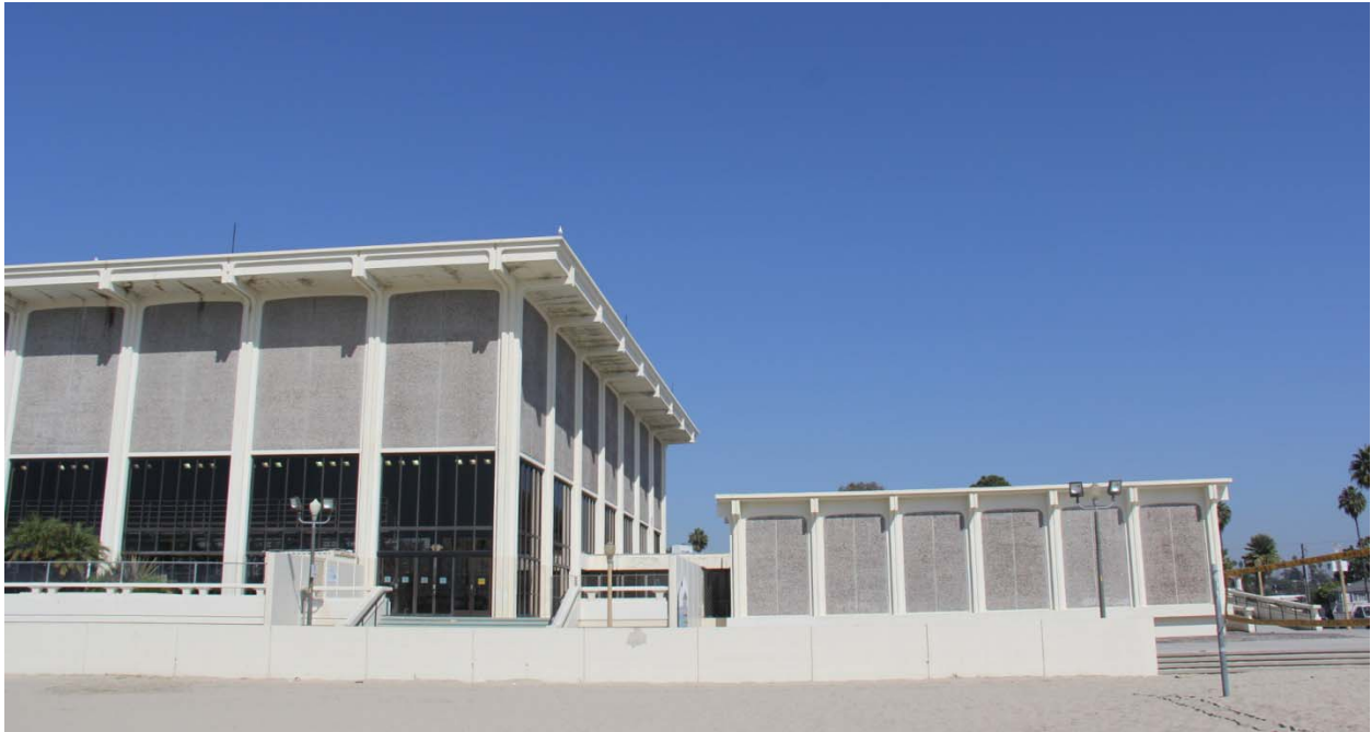
Figure 9 – Locker Building to Natatorium Connection Corridor, South View
