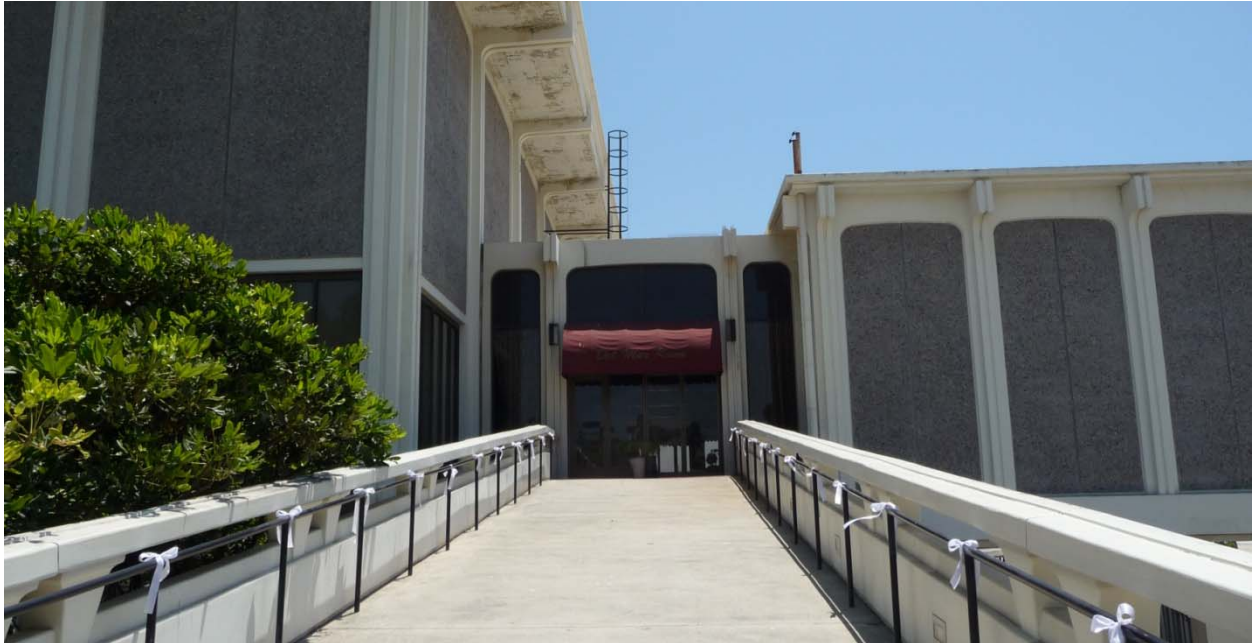
Figure 7 – Ramp at Community Building 2 nd Floor North Entrance
