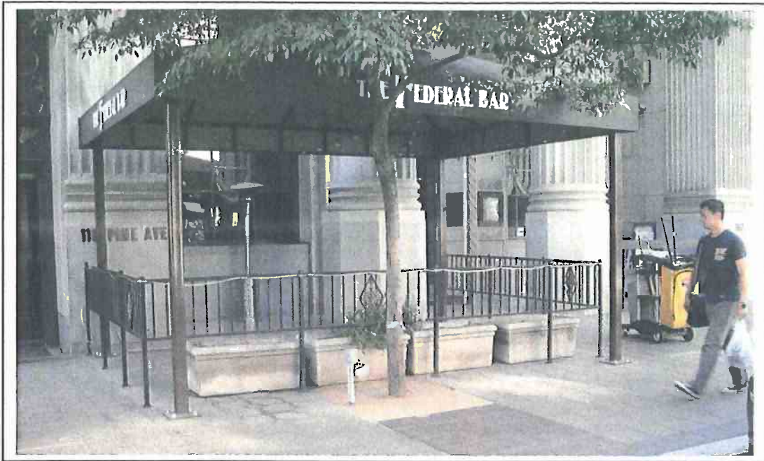
(1) The Federal Bar 102 Pine Ave (View looking East)
