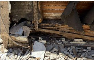
E. It is unknow how many stud walls deteriorate due to moisture, termite, and molding. The visual observation, where studs are exposed, shows a few studs with severe damage. A termite report from a specialized termite company is required to determine which stud wall needs to be replaced.
