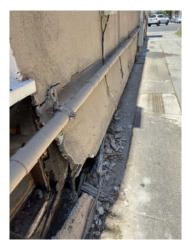
B. The exterior of the building has suffered water damage and termite damage is apparent on three sides of the building, the back and two longer side walls. As a result, the exterior stucco finish is detached from the wood framed walls and buckled.
