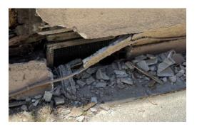
G. This building is supported on a raised floor foundation system. It is unclear if the raised floor joists, beams, posts, and their connections sustain any damage due to water intrusion. The space under the raised floor area was not accessible at the time of observation. All under floor vents do not have curbs to deter rainwater. Water can flow freely into the under-floor areas.
