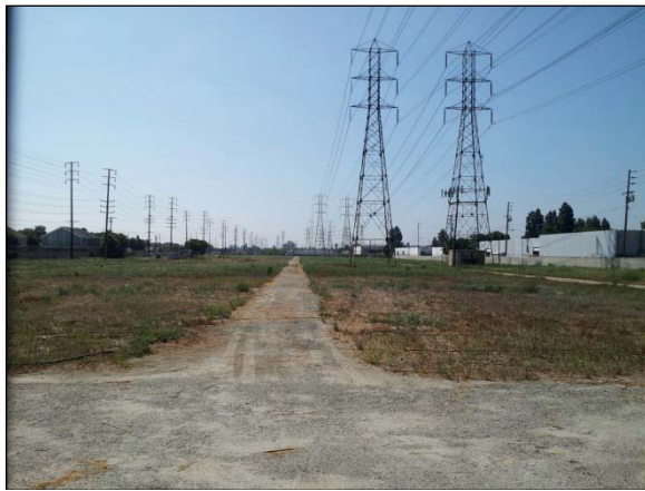
Underutilized right-of-way in Paramount
