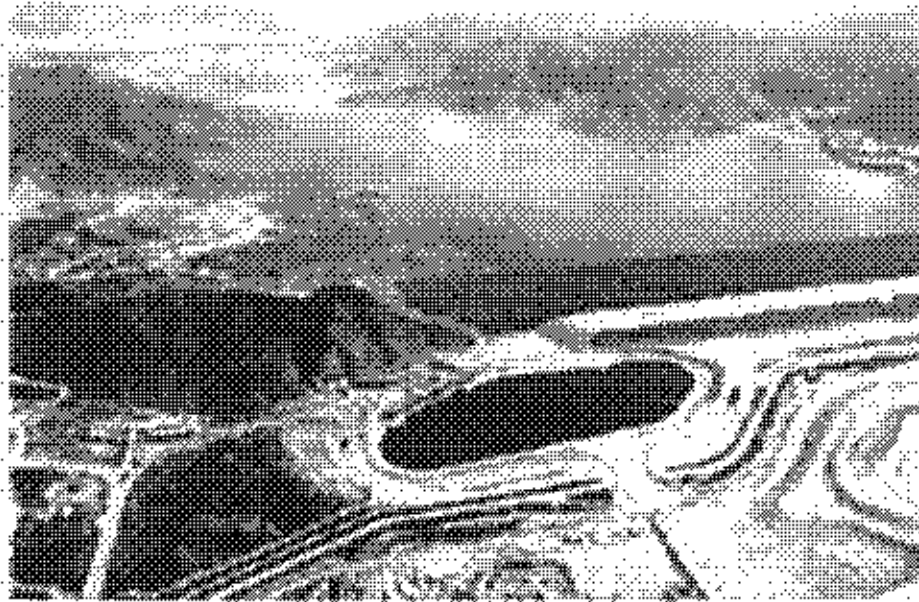
Figure 6: Aerial view of the Diamond Valley Lake.
