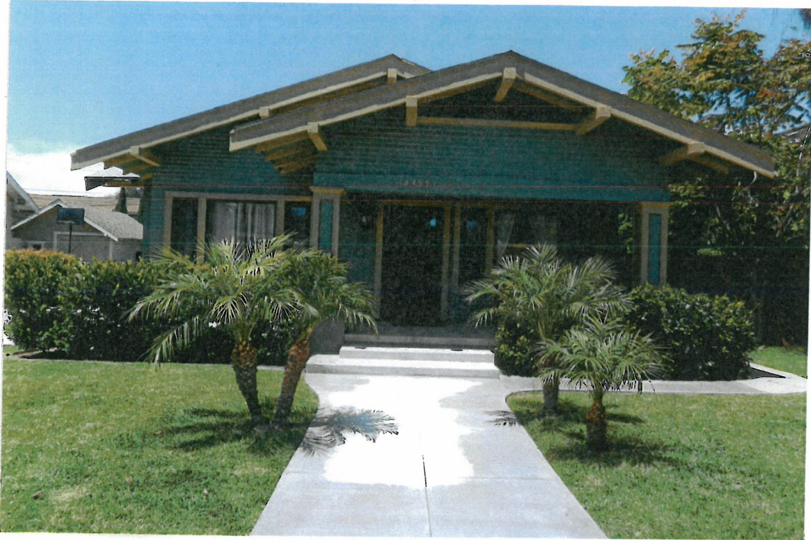
Back House -- Sample of Front Door (Using same windows as front house)
