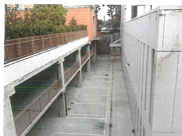
"Moat" along west side looking towards Ocean Blvd.
