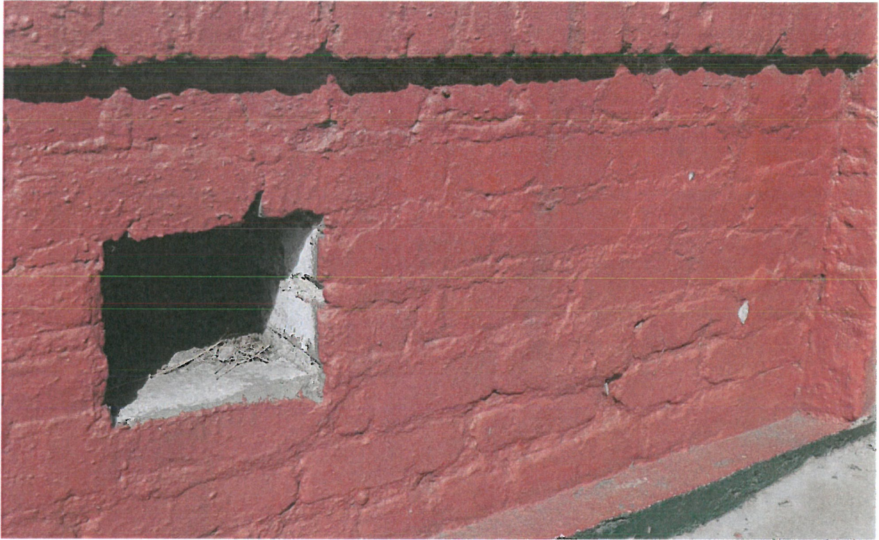
Close-up of Brick Cladding on the Primary Elevation, Photograph: May 2015
