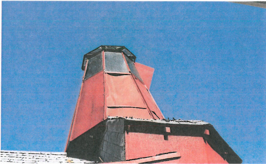
View of Roof-Mounted Spout, Photograph, May 2015.
