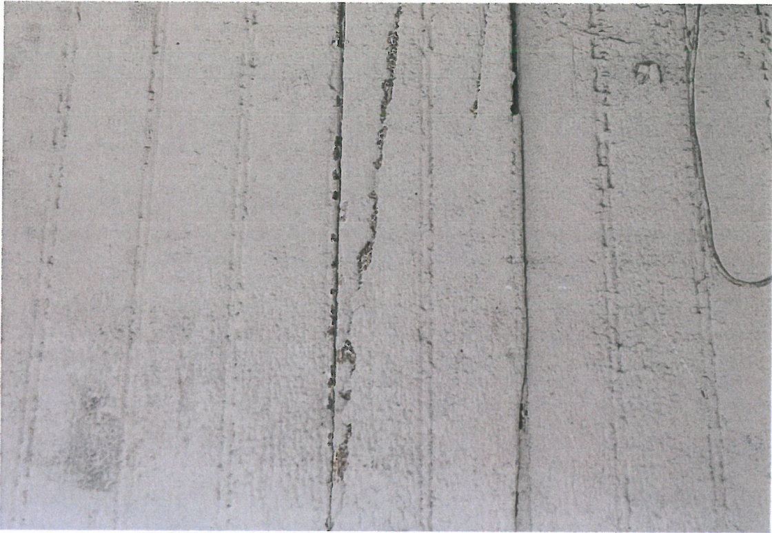
Close-up of Wood Siding on West Elevation, Photograph: May 2015
