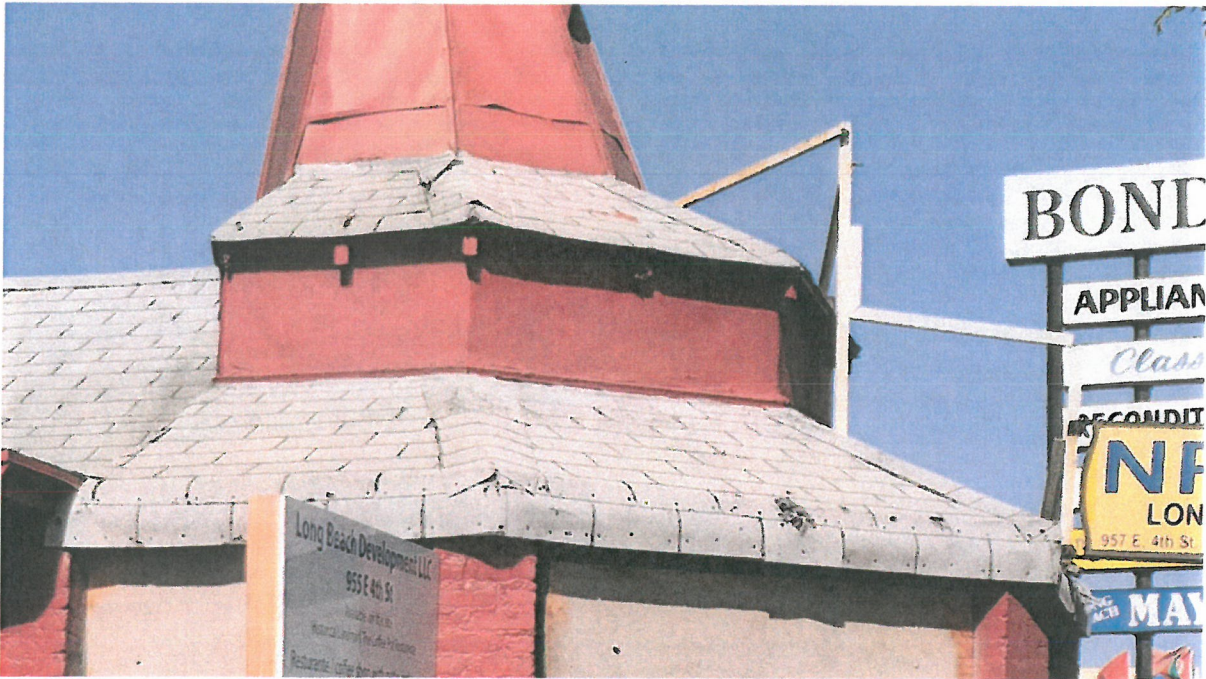
View of Asphalt Roofing on Octagonal Building Portion, Photograph: May 2015
