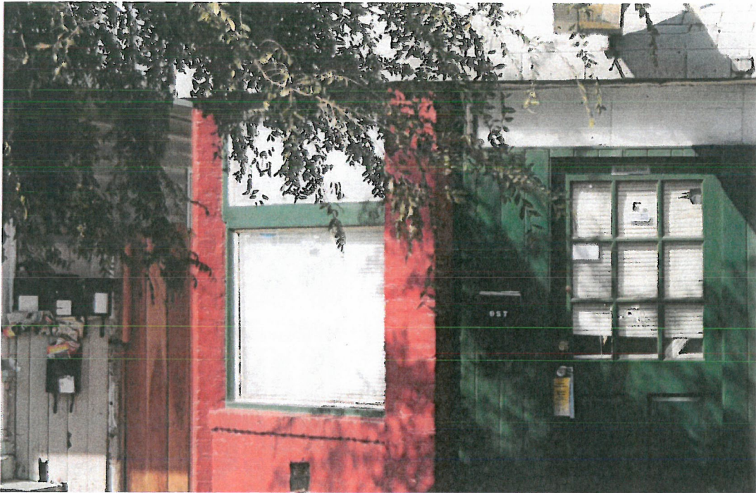
Wood Window on South Elevation, View North, Photograph: February 2015
