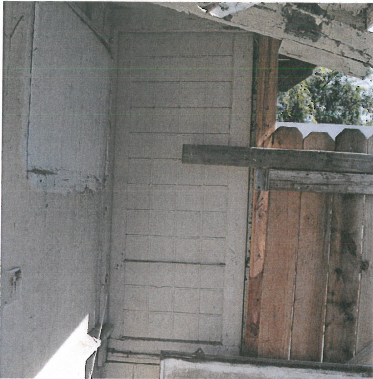
Original Multi-Lite Wood Window on North Elevation, Photograph, May 2015.
