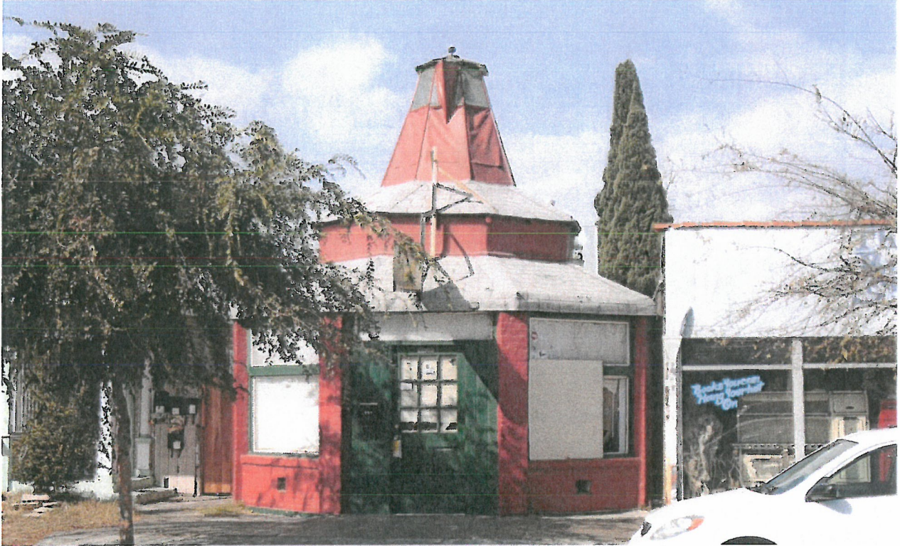
Overview of Octagonal Plan, View North, Photograph: February 2015
