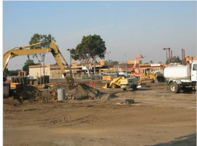
Heavy Equipment at a Construction Site
