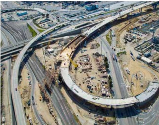
Freeway interchange in Long Beach
