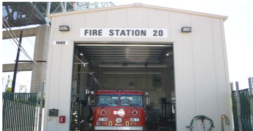
1980 Pier D Street Berth D37 – District 2
