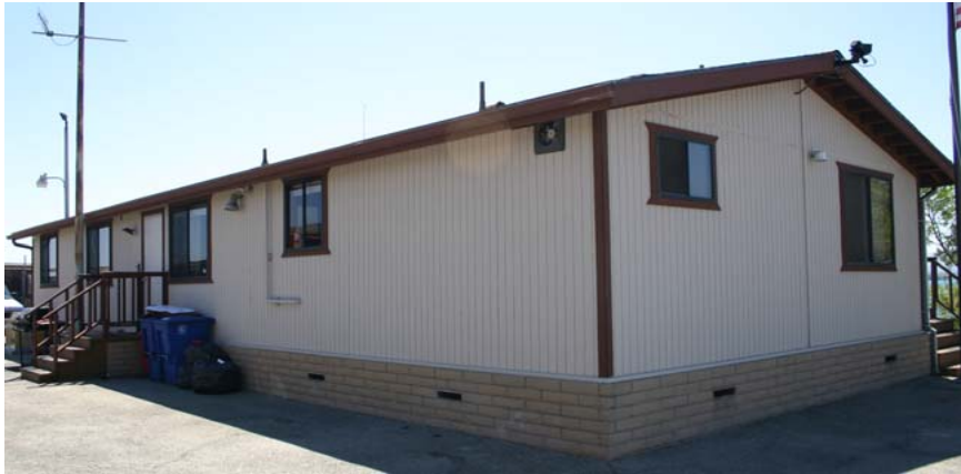
Pier F Berth F202 – District 2
