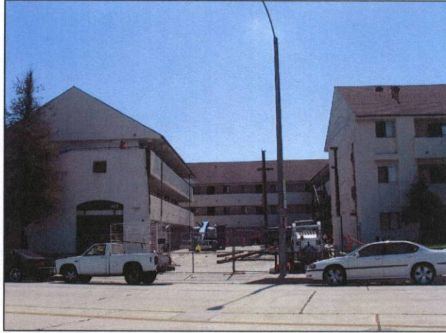
30 Affordable Units - Construction Underway
