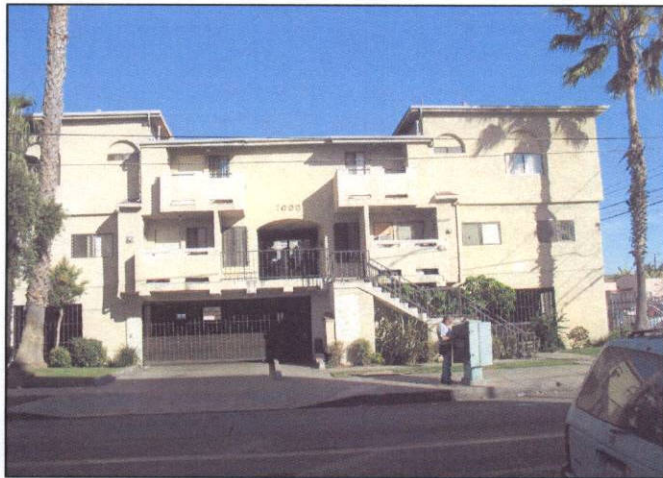
19 Affordable Units - Construction Underway
