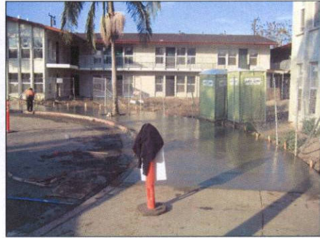
24 Affordable Units - Under Construction
