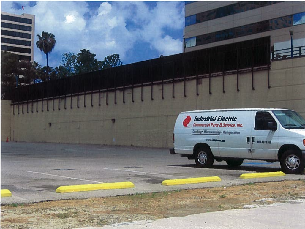
Subject's east property line, retaining wall for Salvation Army Office Building
