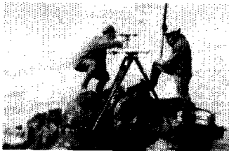
/// Taking Measurements Working under rugged conditions with only basic tools, early Coast Survey teams laid the foundation of knowledge about the nation's coastlines. In this 1921 photo, surveyors in Southeast Alaska take coastline measurements.
