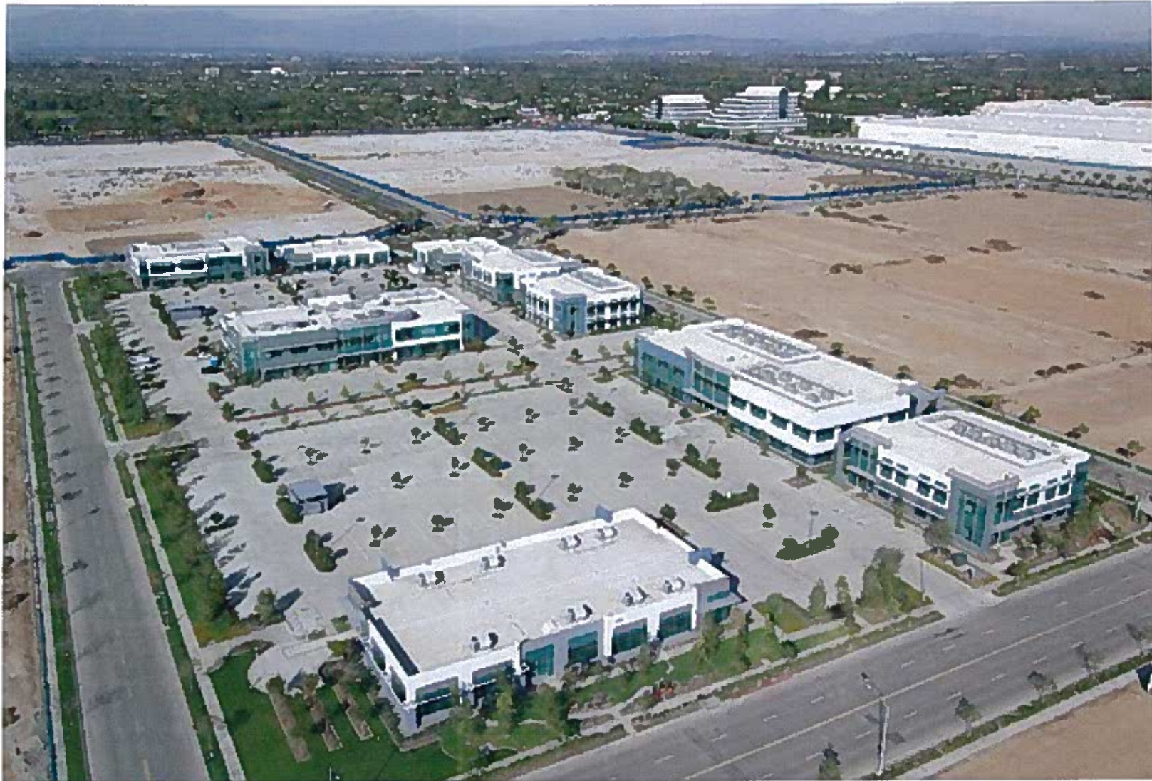
Office Park Completed Southwest of Roundabout
