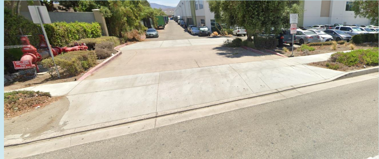
Driveway with sidewalk at the back
