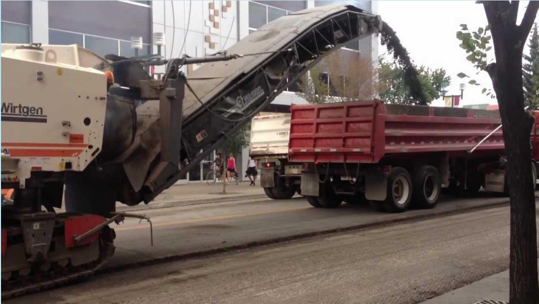
Grinding of road surface
