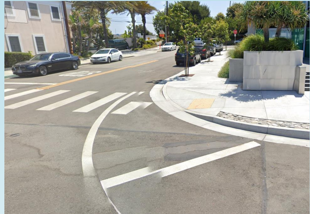
Single directional curb ramp (Case A)
