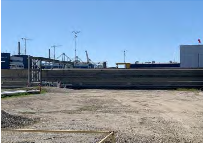
Figure 2-4. Project Site – View Looking West
