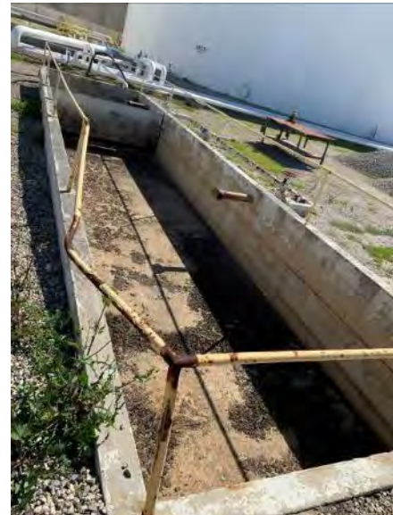
Figure 2-5. Oil/Water Concrete Separator Sump (to be demolished)
