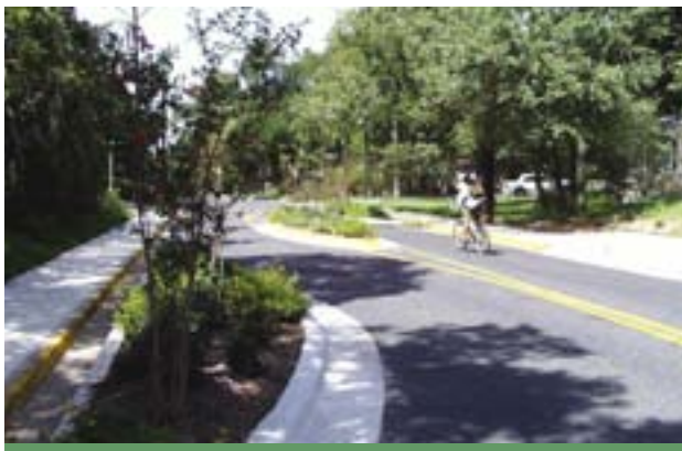
Image 4.8 An example of a chicane from Austin, TX.
