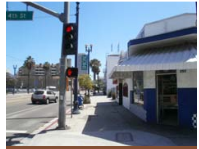
Figure 2.24 A fully-actuated traffic signal at the intersection of Pacific Avenue and 4th Street.
