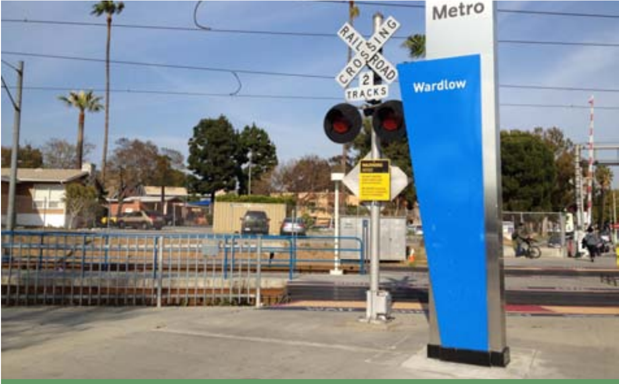
Figure 5.68 Existing Blue Line Wardlow Station.
