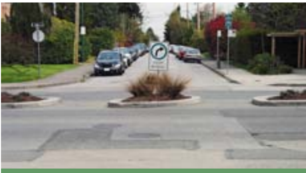
Image 4.7 Diverter - Vancouver, BC Photo: Richard Drdul.
