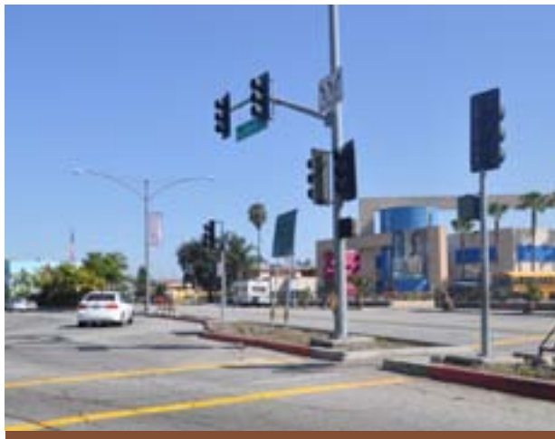
Figure 2.23 Signalized intersection with a pedestrian refuge at Martin Luther King Jr. Avenue.
