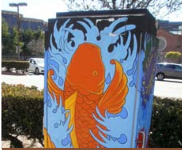
Figure 2.42 Painted utility boxes installed as part of a City-sponsored improvement program.
