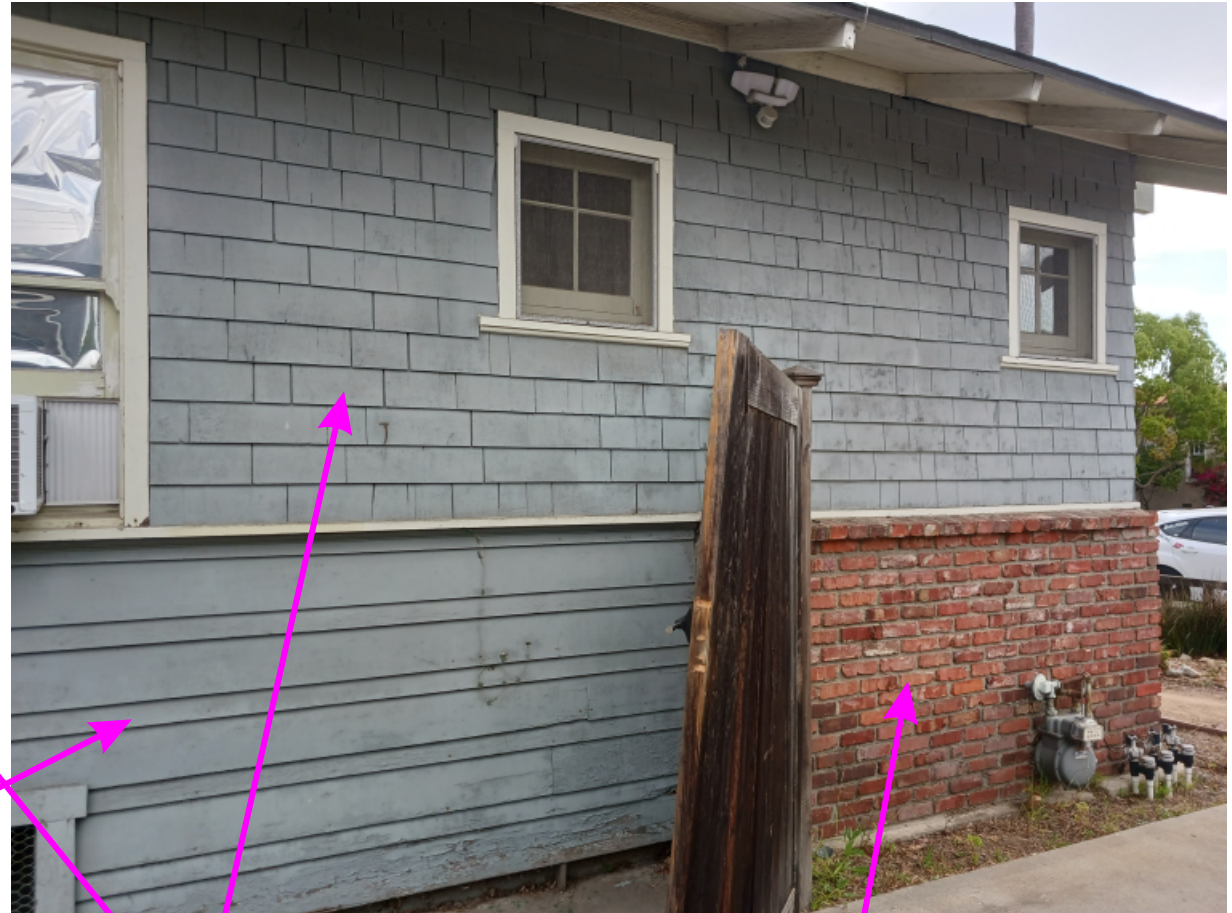
SHINGLE SIDING ORIGINAL MATERIAL
