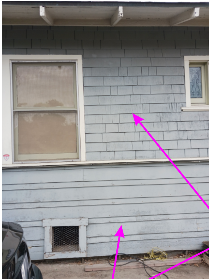
HORIZONTAL SIDING ORIGINAL MATERIAL
