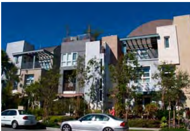
Example of low-rise project with massing and materials that delineate individual units, entrances and roof gardens.
