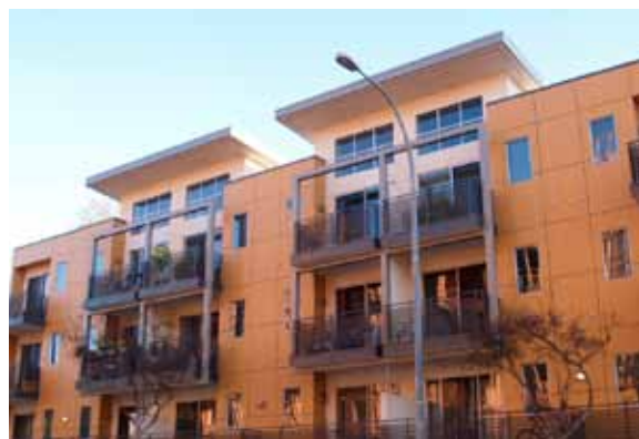
Example of reinforced fiber cement panels integrated in a low-rise residential project.
