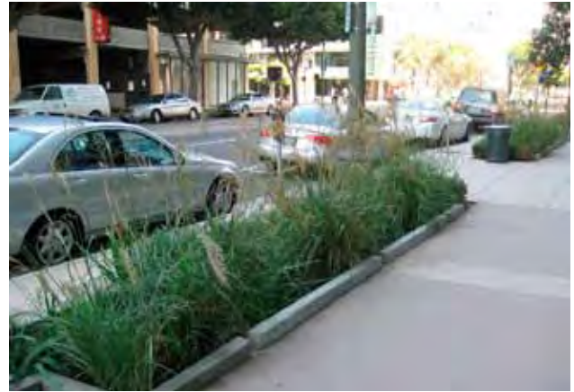
Parkway planting shall be set back 18 inches from the curb to allow for easy access to parked vehicles.
