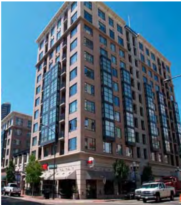
Example of high-quality materials used on a new mid-rise building that exhibits a classic base, middle and top composed of more substantial material and storefront details at the pedestrian level, plus inset balconies and a variety of window types.
