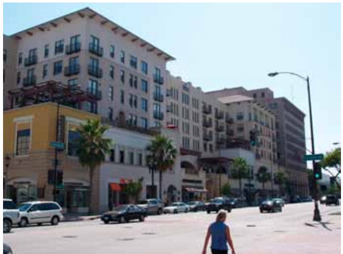
Stepbacks and variation in massing and materials break down the scale of this mid-rise urban infill project. The lower two stories reflect the scale and texture of existing buildings in the neighborhood.
