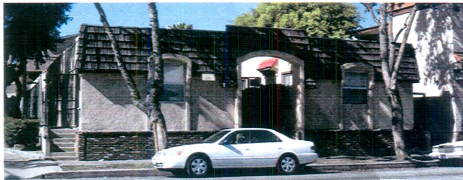
Photo 2: 1027 Redondo Avenue site
