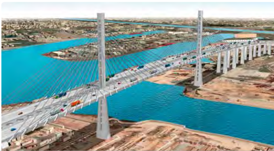
Gerald Desmond Bridge replacement.
