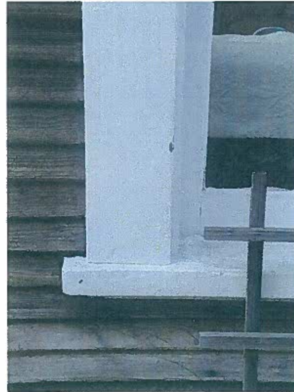
Existing typical window sill
