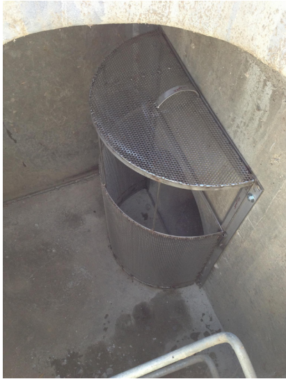
Figure 5-4 A Catch Basin Insert. The 5 mm mesh and inlet at the top allows some trash particles to flow through to avoid flooding problems. Photograph courtesy of StormTek
