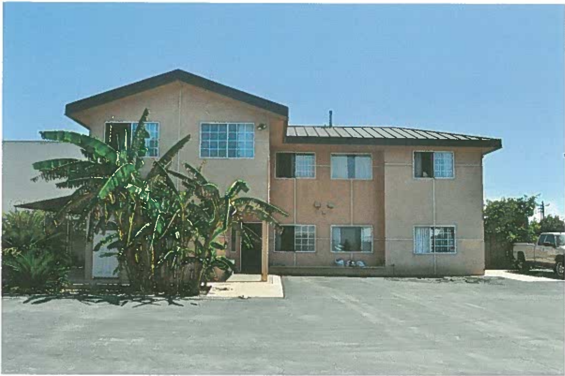
Front Elevation (facing North) of existing 2170 West Esther Street Building
