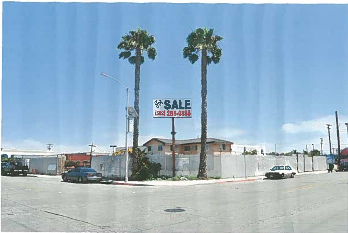
View of Existing 2170 West Esther Street Site (facing North West) taken from North West corner of intersection @ West Esther Street & Judson Avenue
