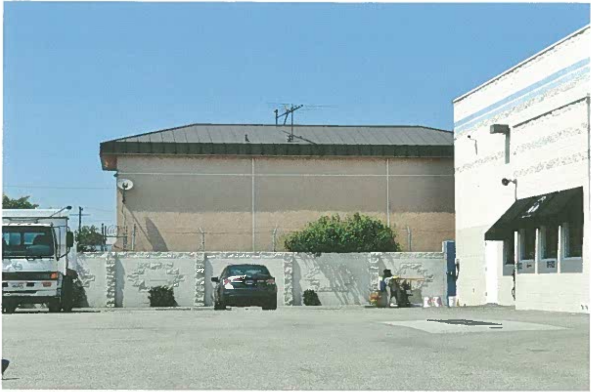
Rear Side Elevation (facing South) of existing 2170 West Esther Street Building
