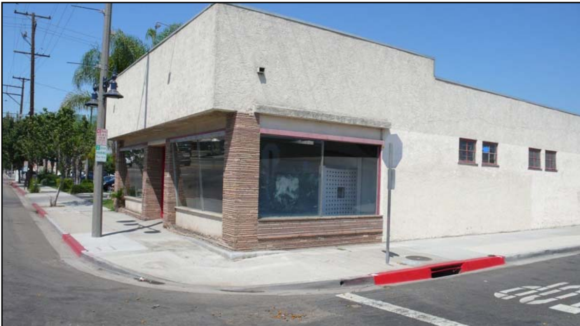
Photo 4 - 635 E. South Street, southern and eastern elevations.
