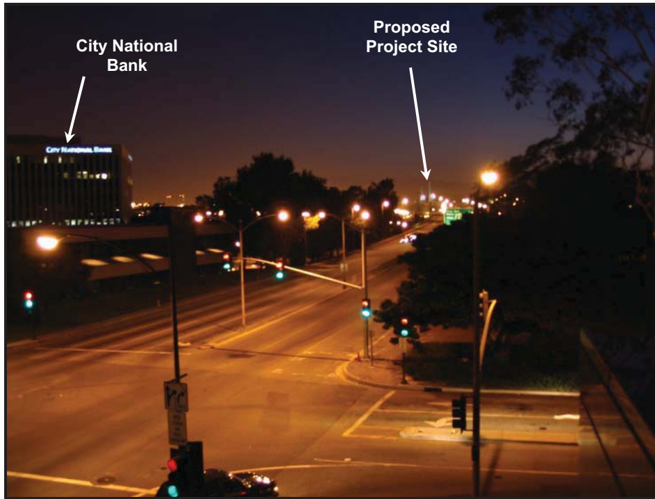
Exhibit 2.1.7-19 Viewpoint 4B – Nighttime Simulation of the Proposed Project (View to the West from Downtown at the Long Beach Hilton)
