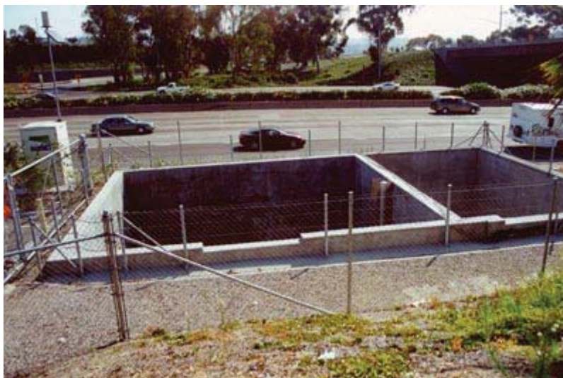
Exhibit 2.2.1-5 Typical Media Filter (Austin Sand Filter)
