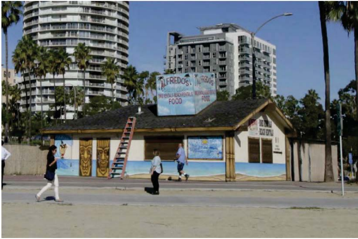
Existing Condition, Northwest View
