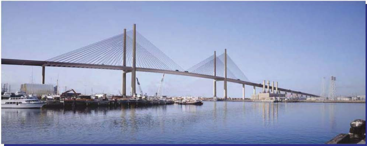
H-Tower with Vertical Legs
