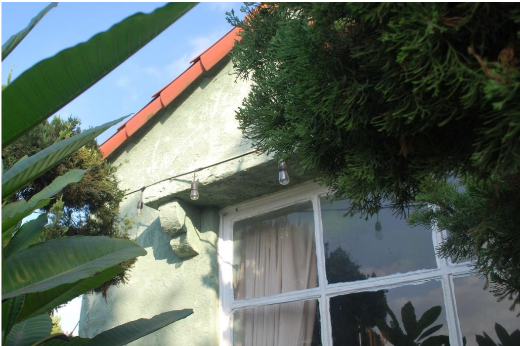
Figure 7 Lintel and Bracket That Likely Have Been Stuccoed Over
