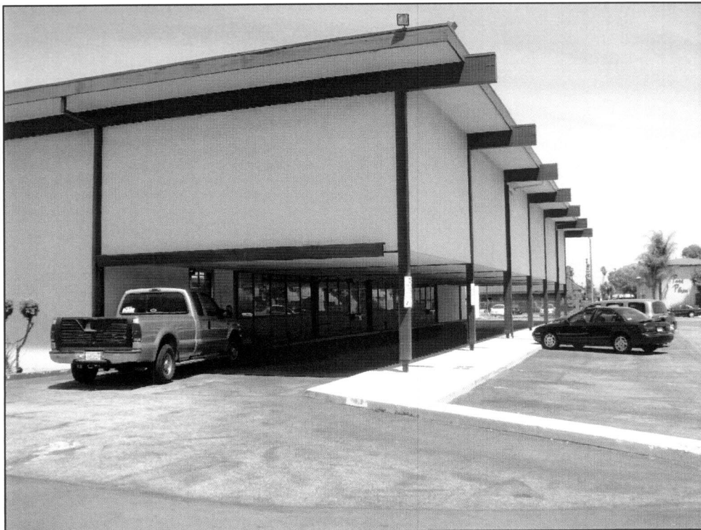
4) View of the extension of the south façade into a drive-in teller lane. Green-painted elements are mostly metal clad in wood showing the primary structural mechanisms. Large trusses extending out from the roof are composite glued wood beams, which were a new innovation in 1962.
