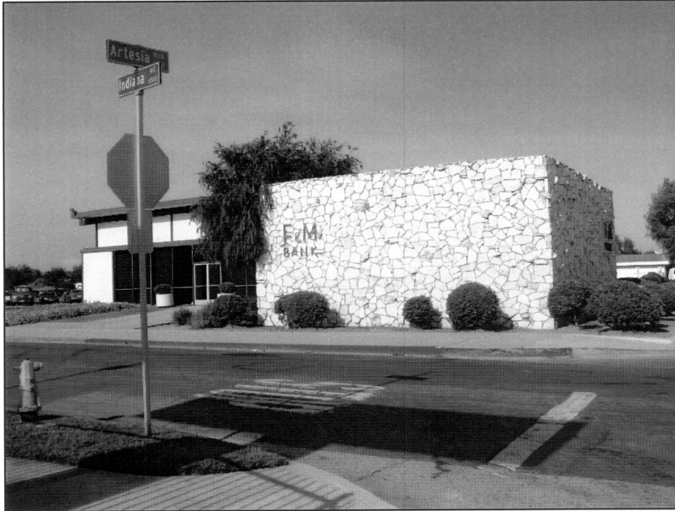
1) East-northeastern elevation of the vault section of the Bank. Note the walls clad in sawn rock typical of post-War commercial styling. Door behind sign originally opened into the Dairy Room.
