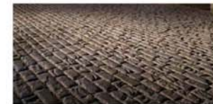
Cobblestone paver driveway apron for reducing speed and warning
