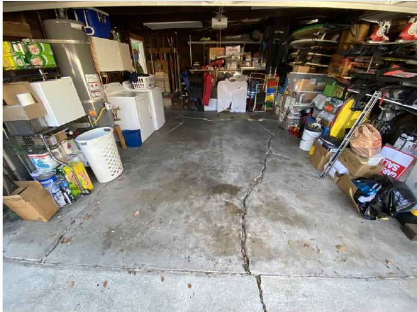
Cracked concrete slab
