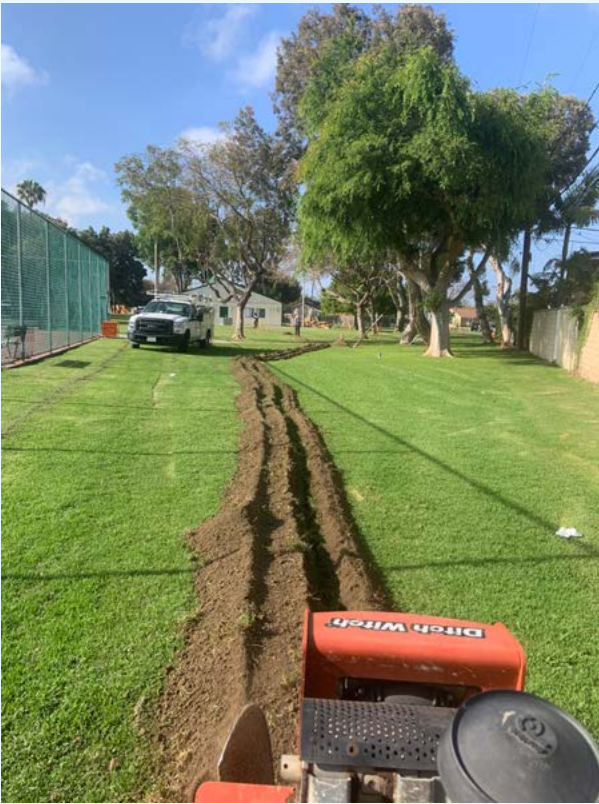
Clockwise from left: trenching for irrigation; Eduardo Magallon wiring up valves; Raul Martinez (left) and Clemente Cerillos help oversee project, Roberto Quinonez (left) and Juan Rodriguez work on wires, Eduardo Magallon and Jaime Sanchez installing mainline.
