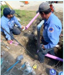
Eduardo (left) and Jaime installing backflow.
