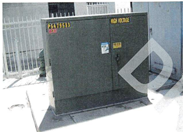
Pad-mounted transformer
