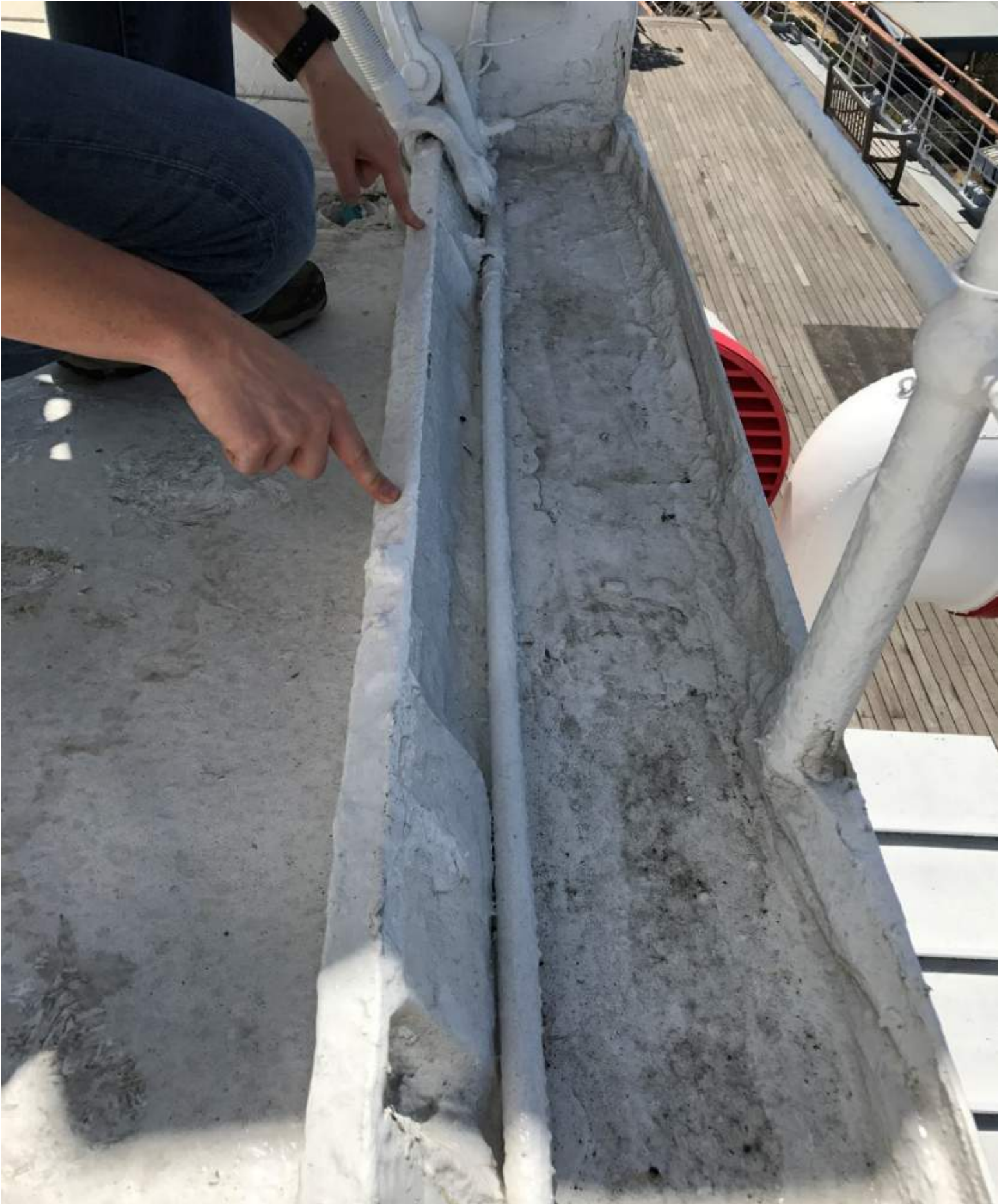
Photo 5 - Existing continuous bent plate in current weatherproofed condition
