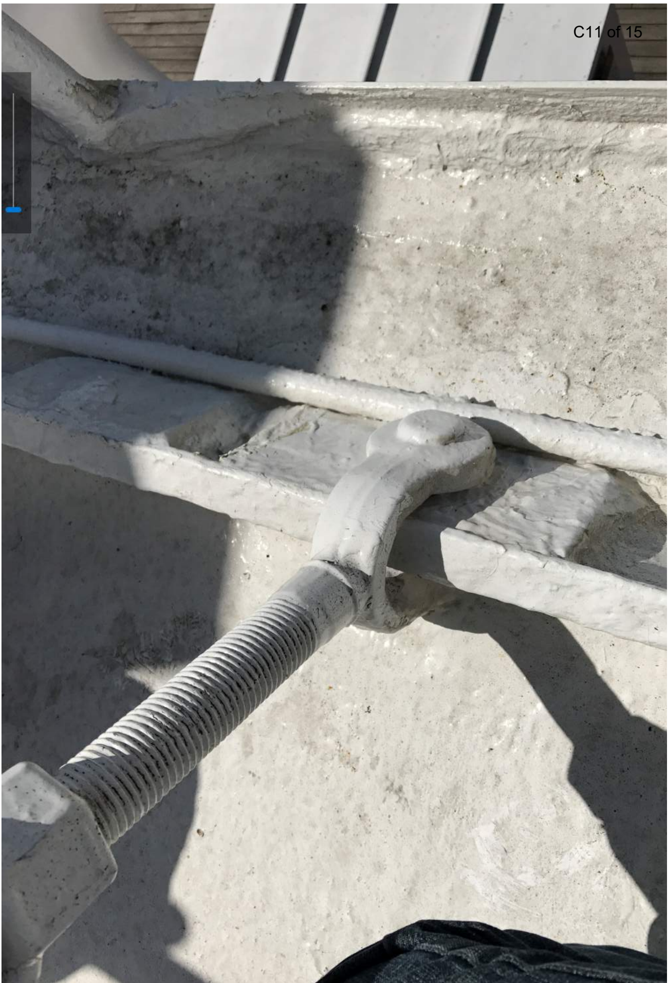
Photo 7 - Rod, clevis, and pin attachment to weatherproofed plates
