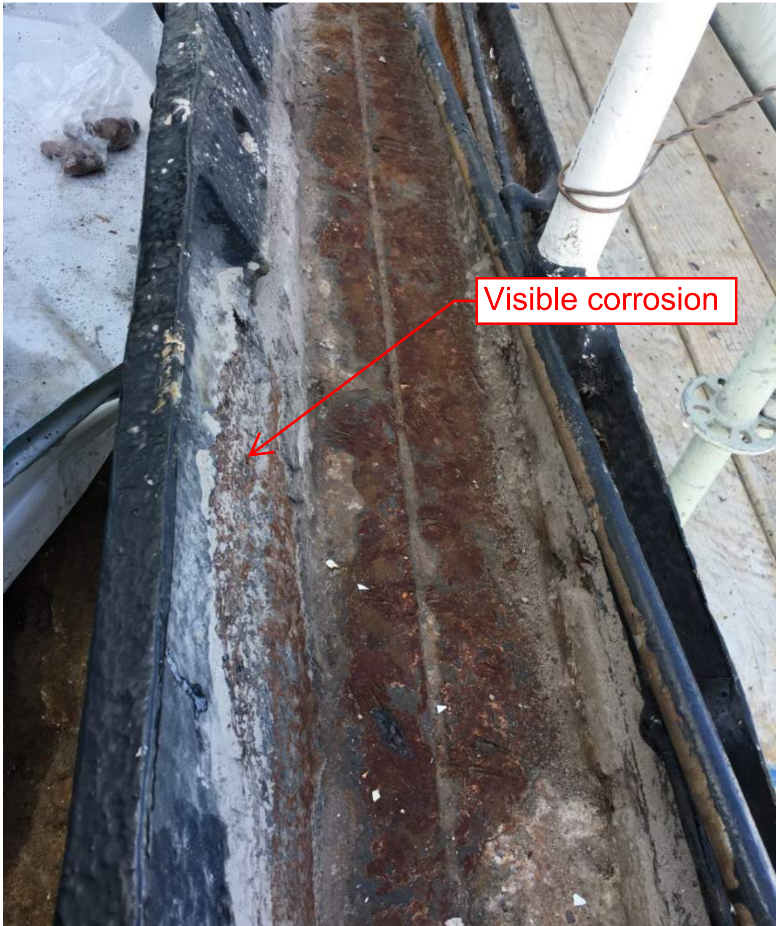
Photo 3 - Existing continuous bent plate corrosion
