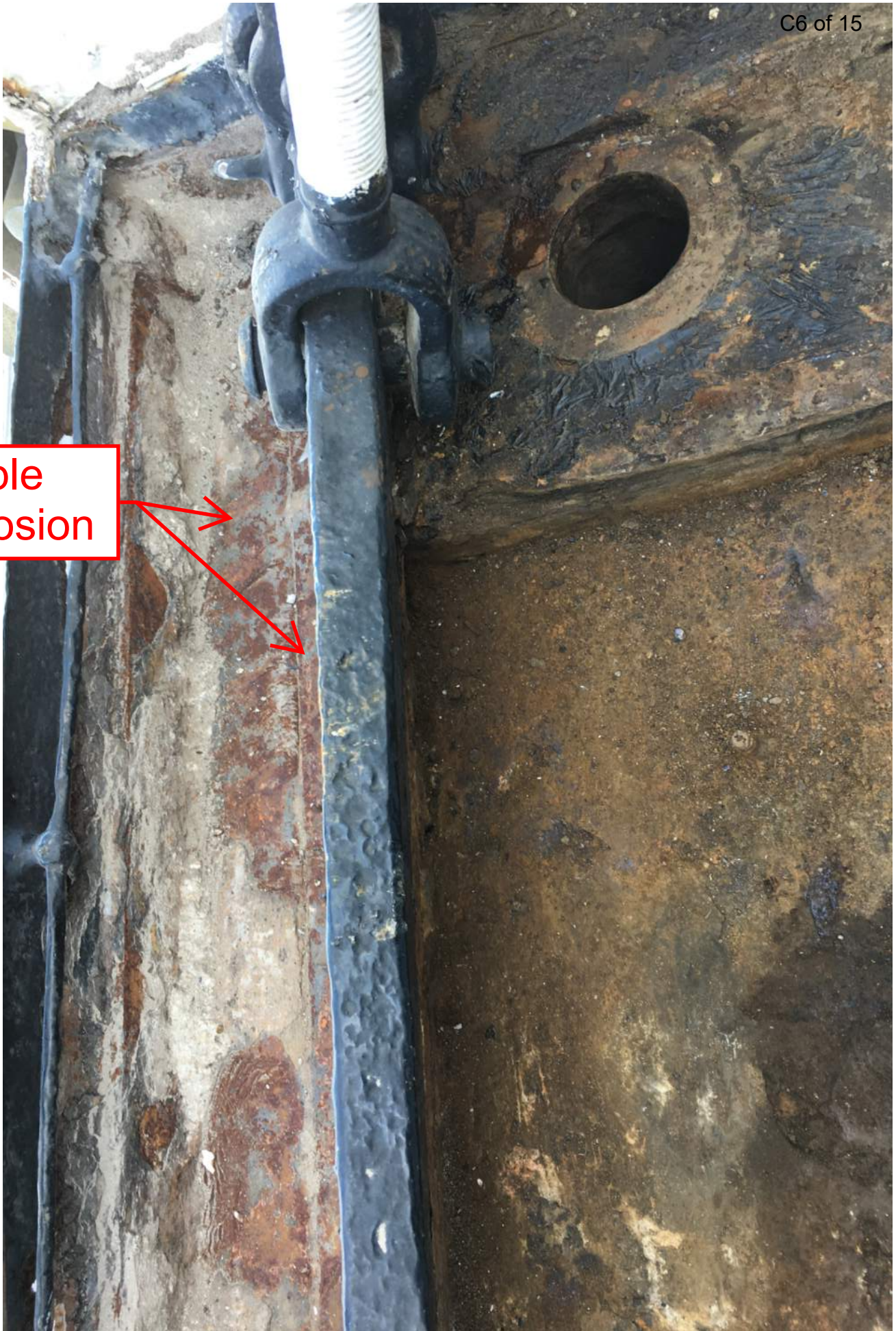
Photo 2 - Existing continuous bent plate corrosion
