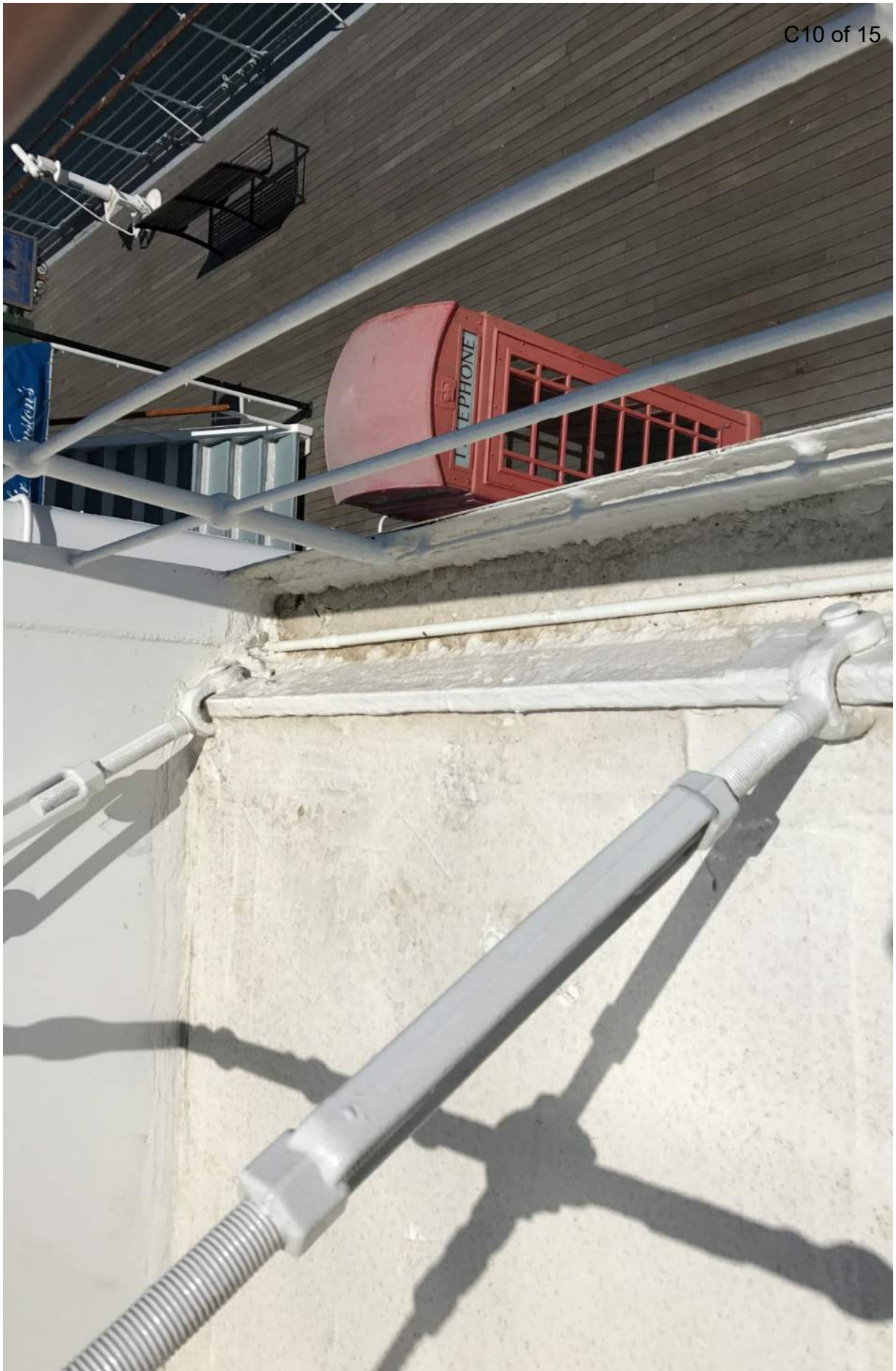
Photo 6 - Existing continuous bent plate in current weatherproofed condition
