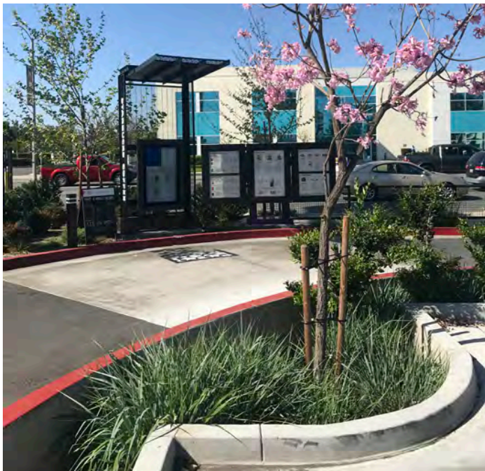
Storm water runoff is collected in planters.
