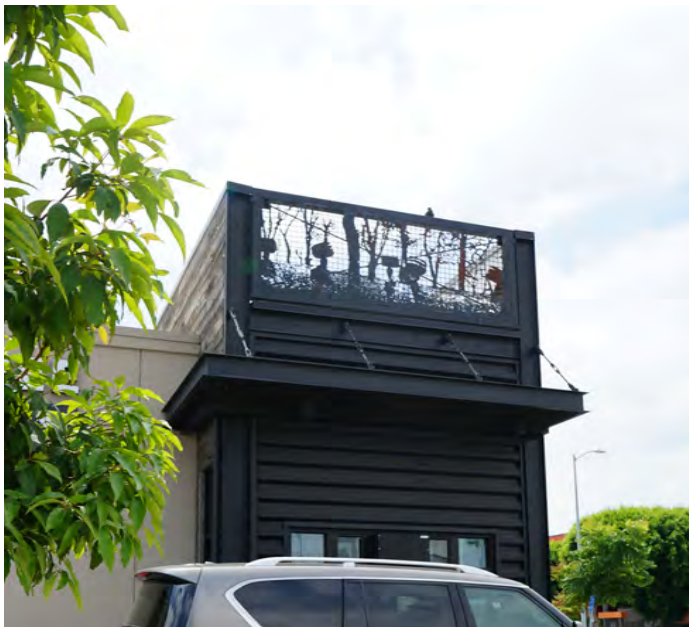
Roof equipment screened in an architecturally compatible manner.
