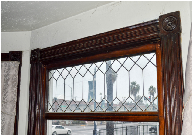
On the first level only, windows have decorative dart and other detailing in the wood window surrounds. Three of these window frames have been painted or varnished (demonstrated through the two images at right) while most are unpainted and sealed (as seen in the left-most image.)
