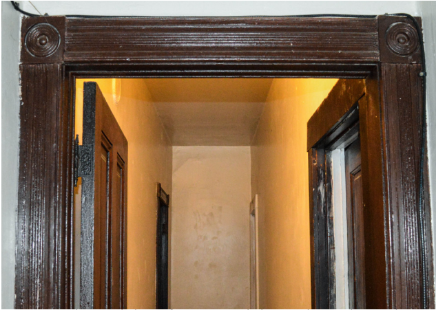
Unpainted wood door frames and doors throughout the first story are in need of repair and restoration.
