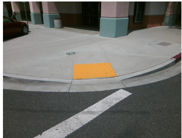
Curb Ramp Detectable Warning Surface
