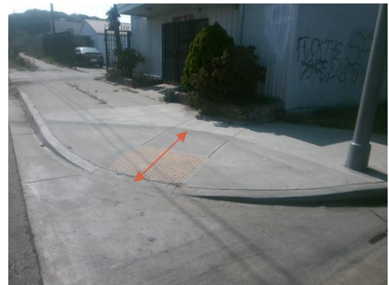
Curb Ramp Run Slope
