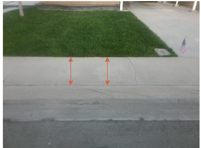
Sidewalk Cross Slope, as depicted by arrows
