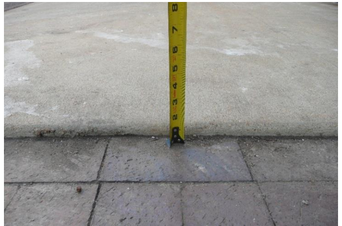
Change in Level at Sidewalk Joint
