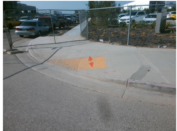
Curb Ramp Cross Slope
