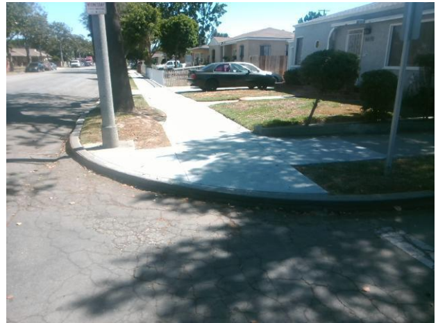
Missing Curb Ramp
