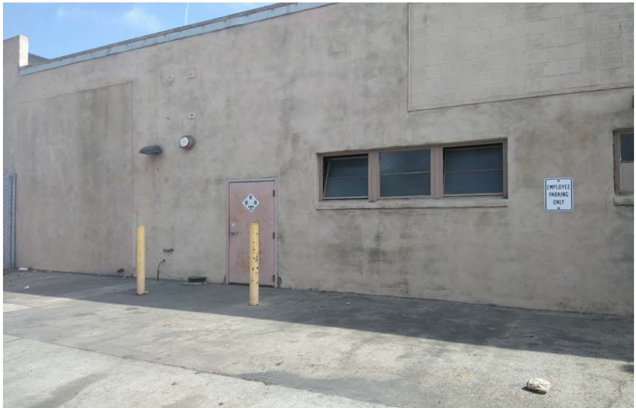
Parking and Side Entrance
