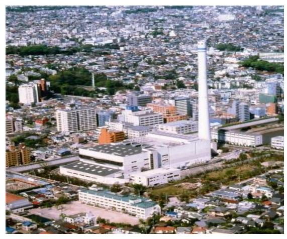
Date Completed: March 1991 Capacity : 300ton/day x 2 lines Power Output : 11,000 kW
