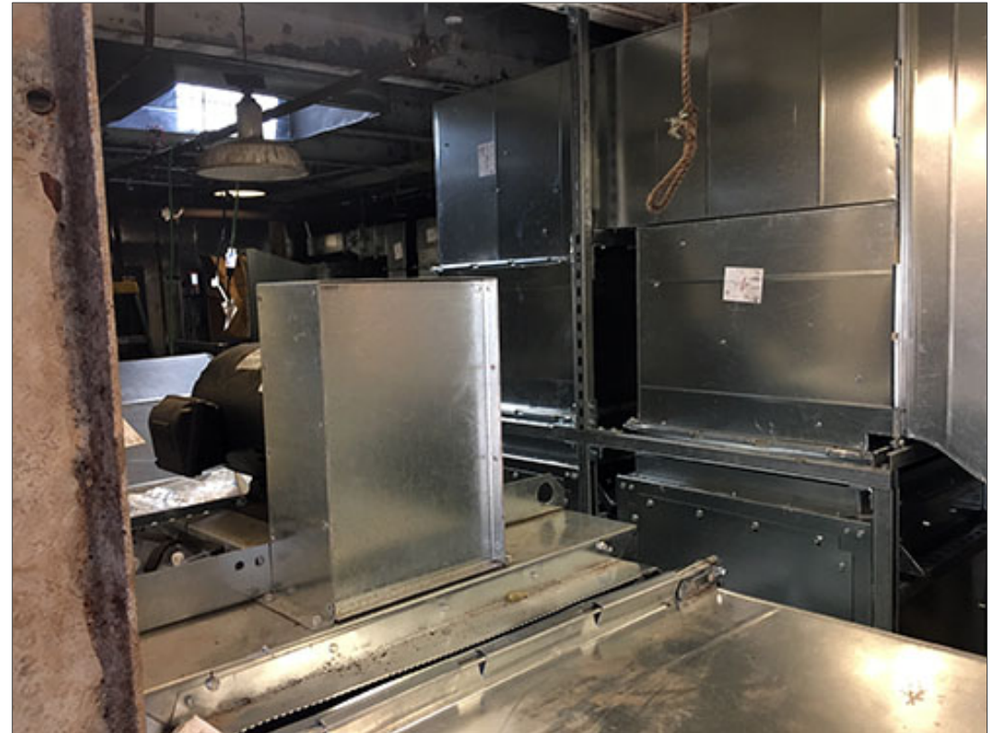
HVAC installation at Frame 200, top of house
