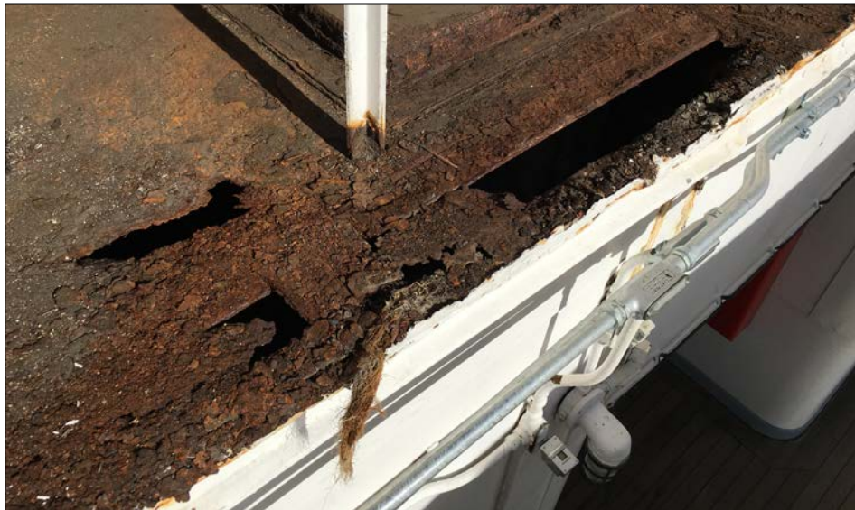
Roof damage and repair/waterproofing on Bridge deck (above Captain's Quarters)
