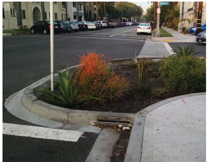
This bioswale helps clean polluted stormwater. - 2nd Street and Orange Avenue.
