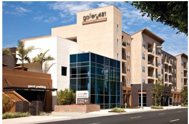
Urban residential apartments.
