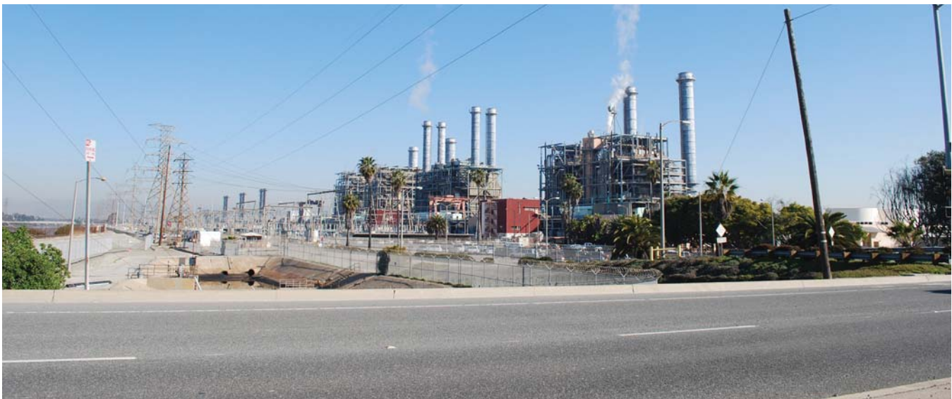
LADWP Haynes Generating Plant in Southeast Area Development and Improvement Plan (SEADIP).
