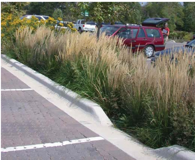
Parking lot bioswales help filter out pollutants.
