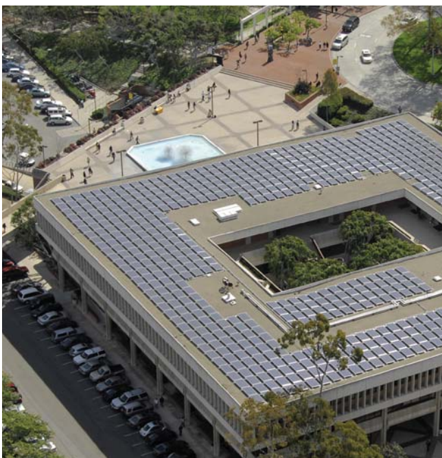
Solar panels on Brotman Hall at CSULB.
