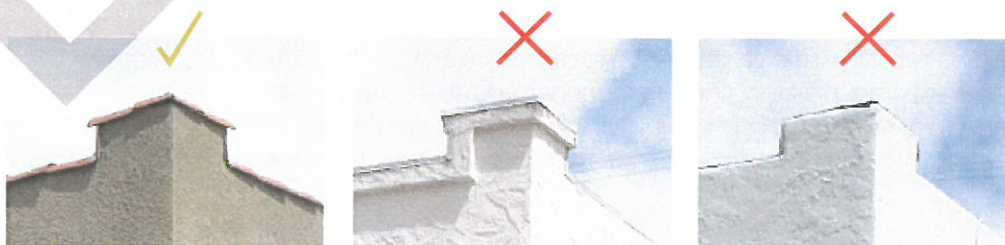
Clay tile coping should remain around a parapet (left); it should not be replaced with metal flashing (center) or removed entirely (right).
