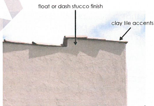
flat roof with parapet walls
