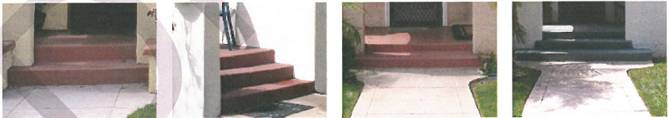
The majority of porch floors and steps within the district are historically appropriate smooth concrete, and may be painted in compatible colors.
