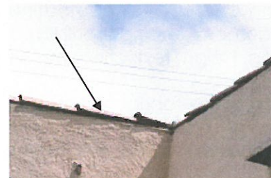
Clay tile coping along a parapet wall.
