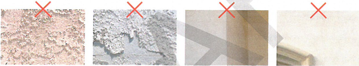
Heavily textured "lace" finish stucco (left) or extremely smooth stucco are equally inappropriate stucco finishes for historic buildings, and should not be applied.
