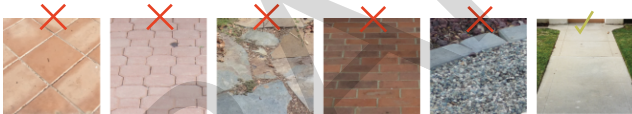
Smooth concrete with scored joints is the recommended material for walkways and driveways.
