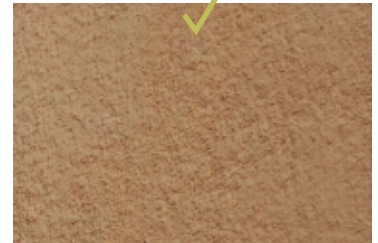
An appropriate float or dash finish stucco has a slightly rough, sandy texture.
