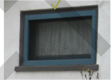
This wood window screen, painted blue, does not detract from the historic window behind it.
